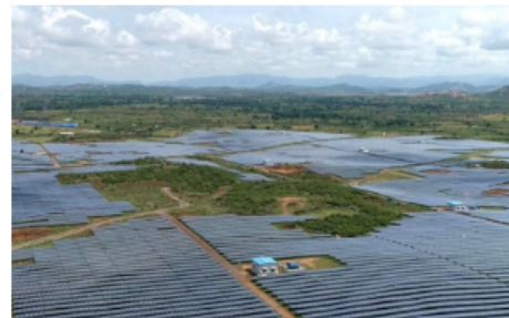
Solar power plant. Source: Tata Power.
