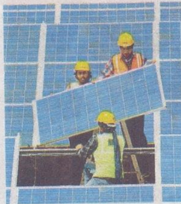
The Aache-gaon project is likely to be commissioned by March 2024. AFP
